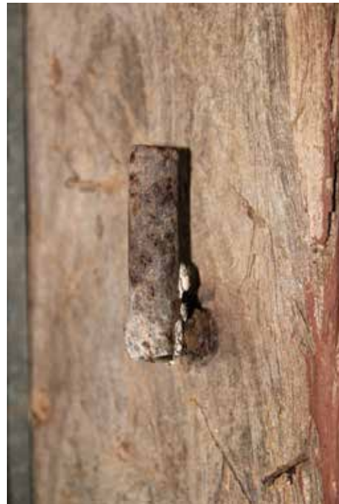
Figure 80 Gudgeon hinge post
