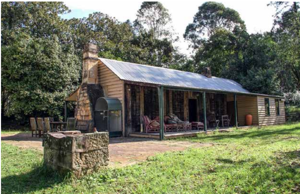
Figure 50 – Rear of cottage in early 2010, prior to connection to inn
