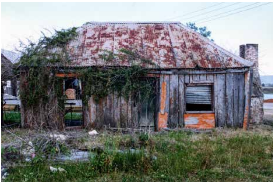
Figure 1 Early slab cottage 4
