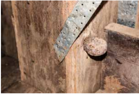
Figure 77 Base of post hinge for door
