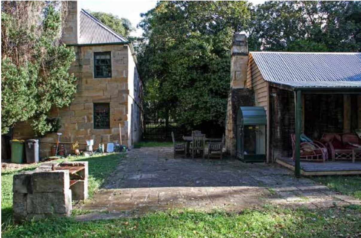
Figure 51 – Rear of buildings in early 2010, prior to construction of connecting room
