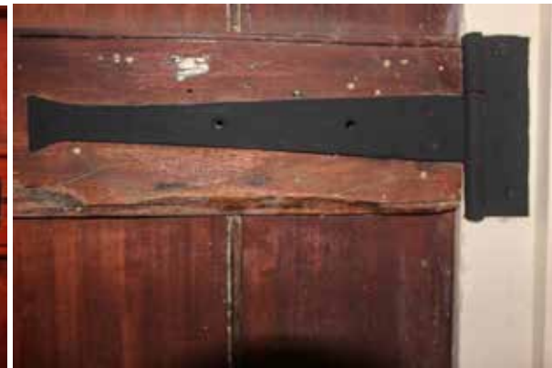
Figure 111 Tee hinge on new ledged door Figure 112 Tee hinge on old ledged door
