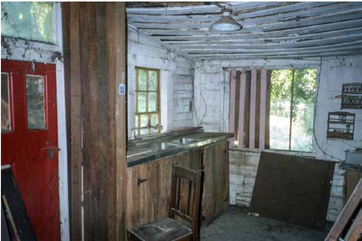
Figure 43 – Another view of original kitchen, including new bench and sink
