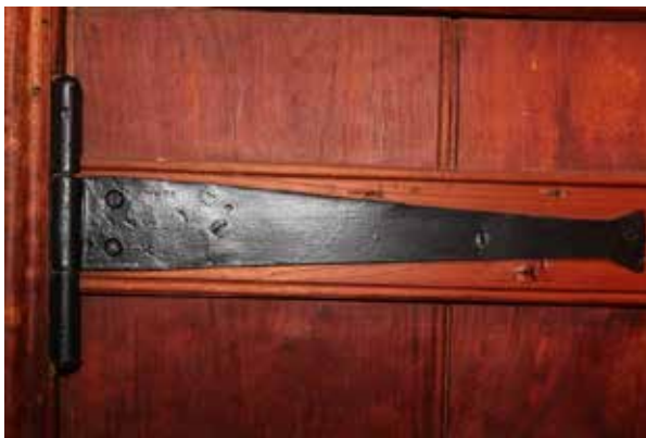
Figure 111 Tee hinge on new ledged door Figure 112 Tee hinge on old ledged door
