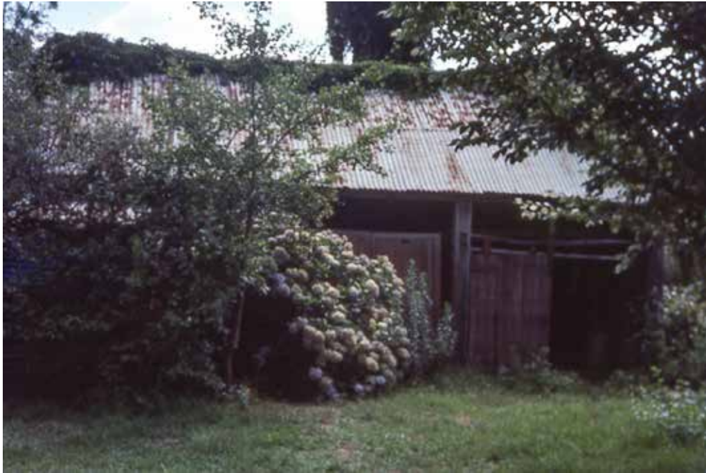
Figure 71 – West side of barn in 1975
