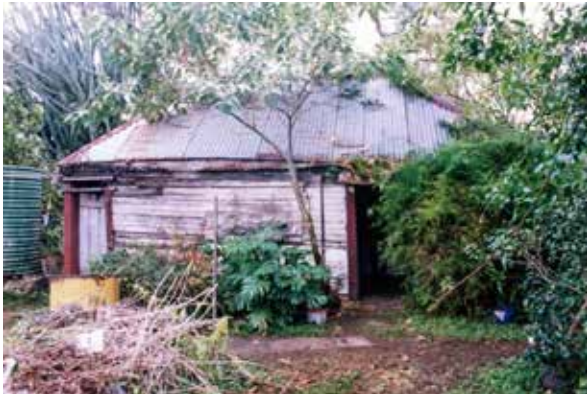
Figure 2 Eastern elevation of cottage 7
