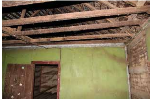
Figure 18 Interior of original slab section
