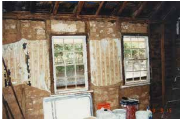
Figure 5 Inside during restoration
