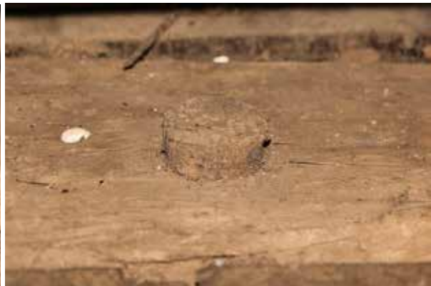
Figure 76 Timber peg joint
