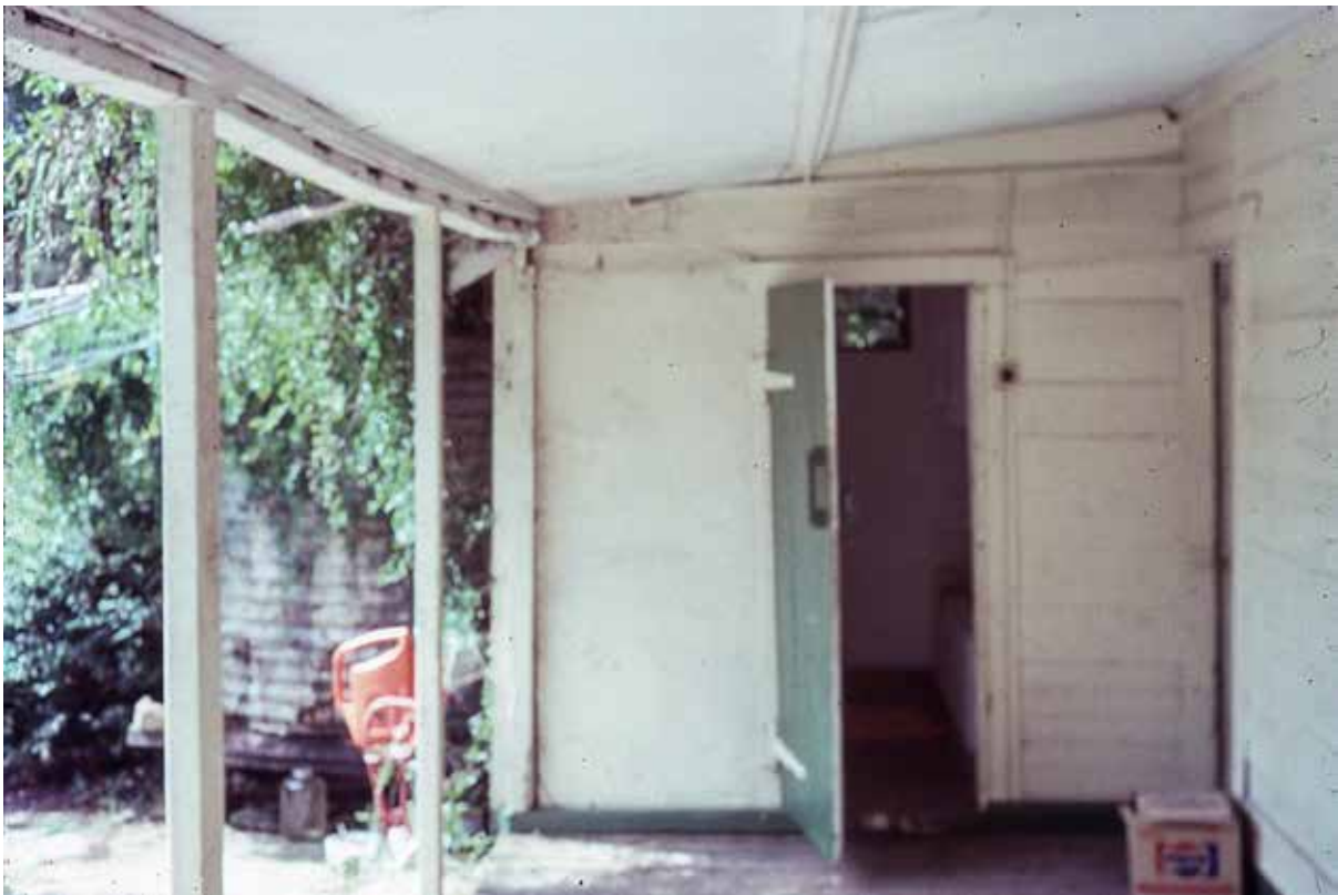
Figure 35 – Rear verandah, looking to bathroom
