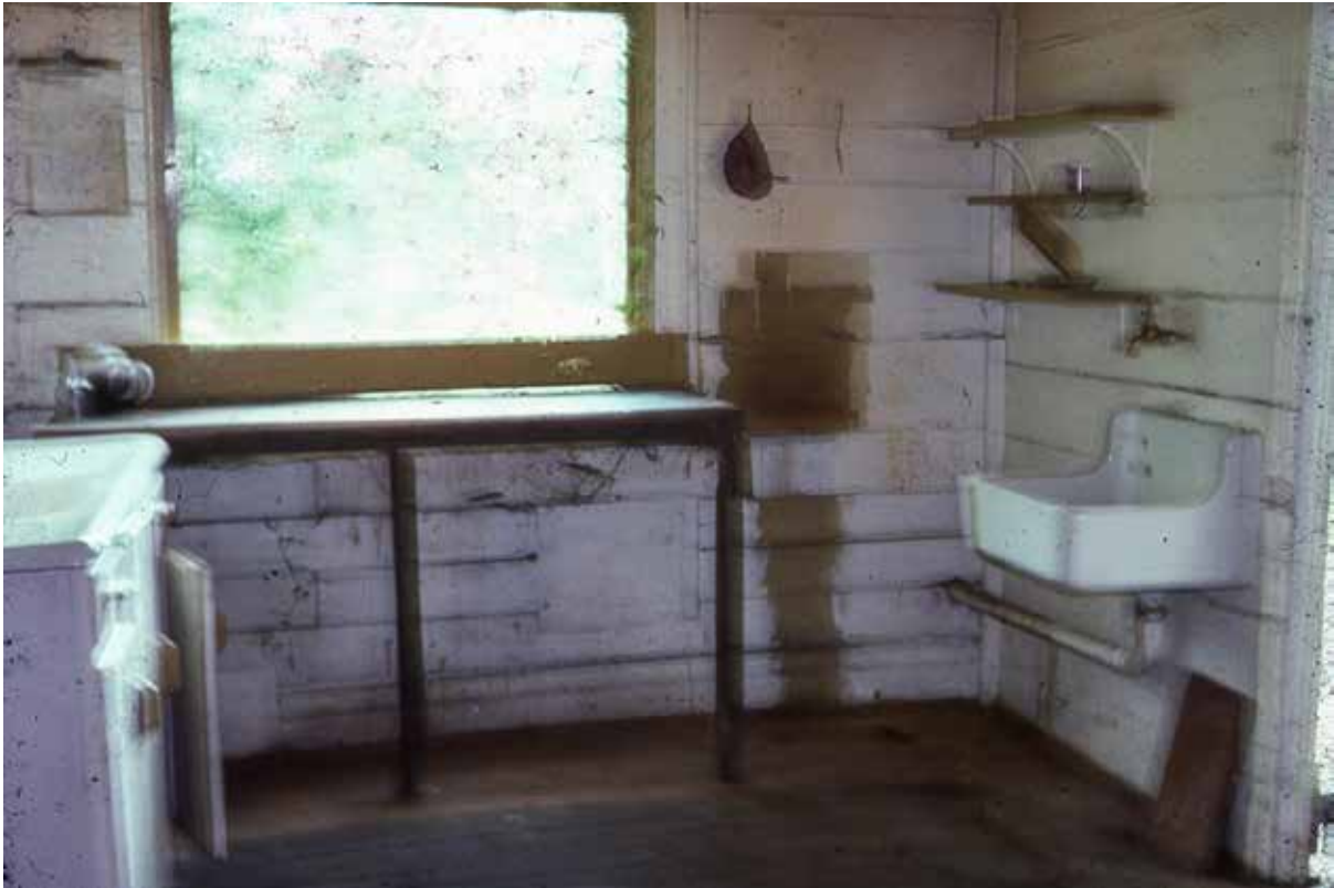
Figure 40 – Inside original kitchen - 13 - 1975
