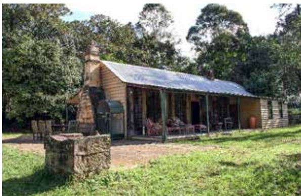
Figure 4 Rear of cottage prior to extensions
