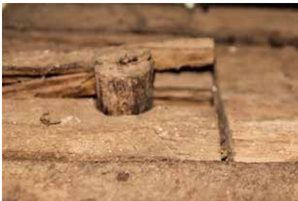
Figure 75 Timber peg joint
