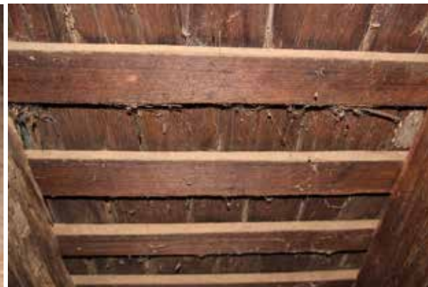
Figure 84 Underside of shingle roof
