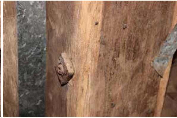
Figure 78 Screw on other end of hinge bar
