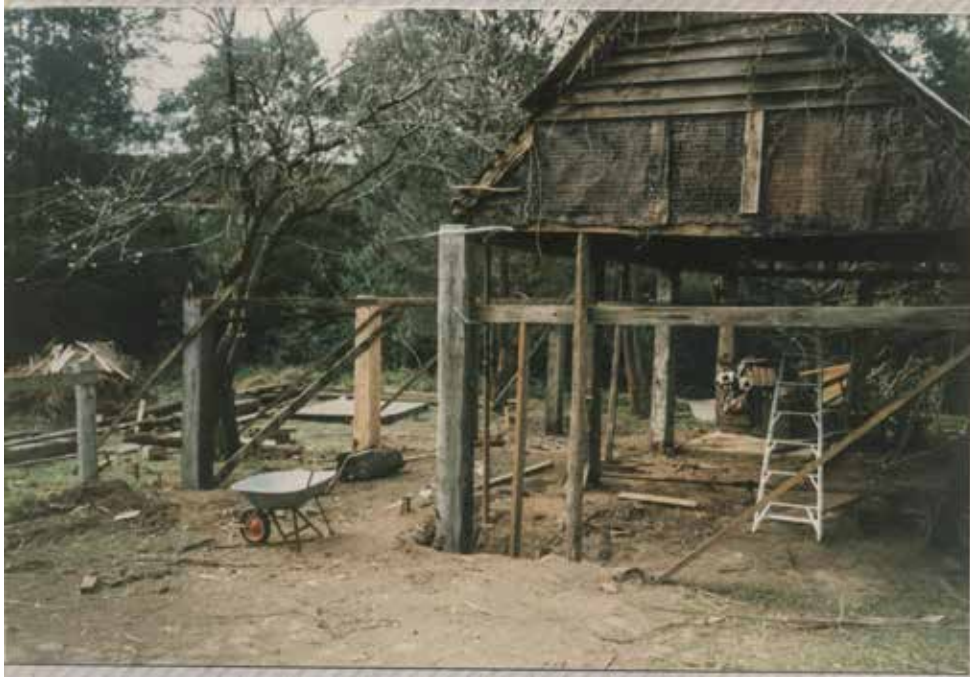
Figure 73 – Barn reconstruction in 1987
