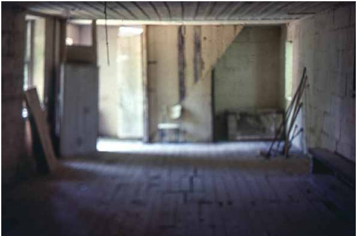
Figure 64 Inside ground floor, looking to stairs - 1975
