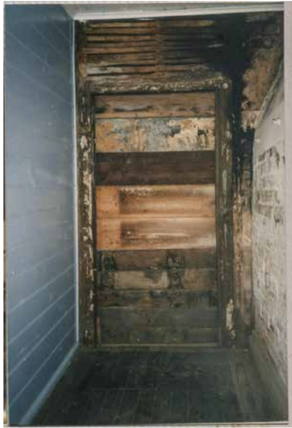
Figure 49 – Original Door 22 in Room C
