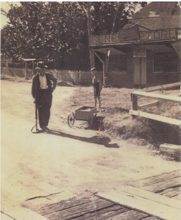
Figure 17 Wheeny Creek Bridge with Home Guard
