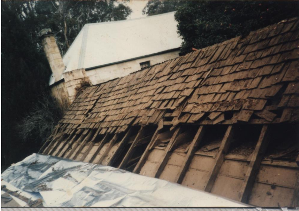
Figure 60 Roof over Rooms 1 & 2, after removal of iron sheeting
