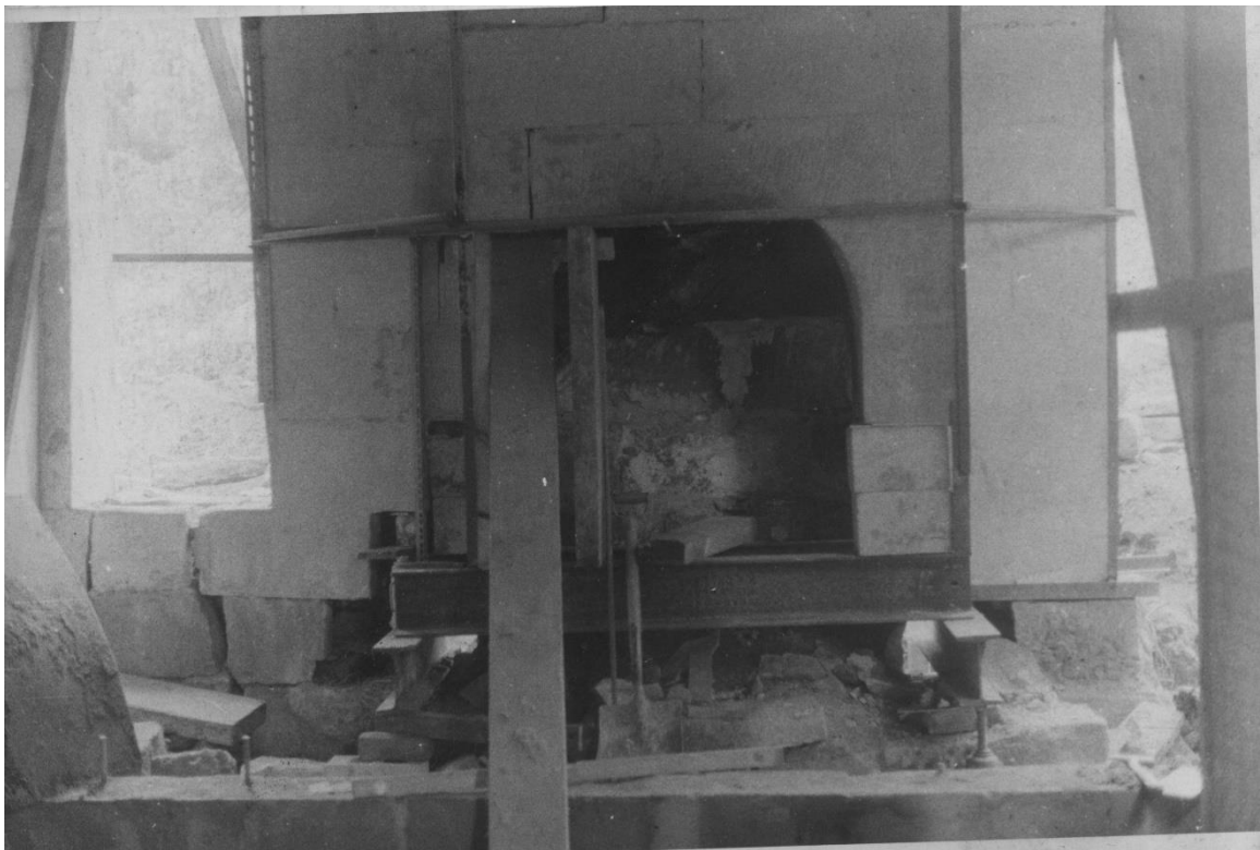
Figure 49 West Wall; Fireplace and wall temporarily supported by steel beams
