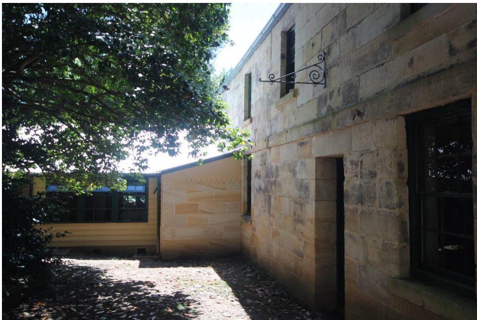
Figure 89 Front courtyard with infill stone wall
