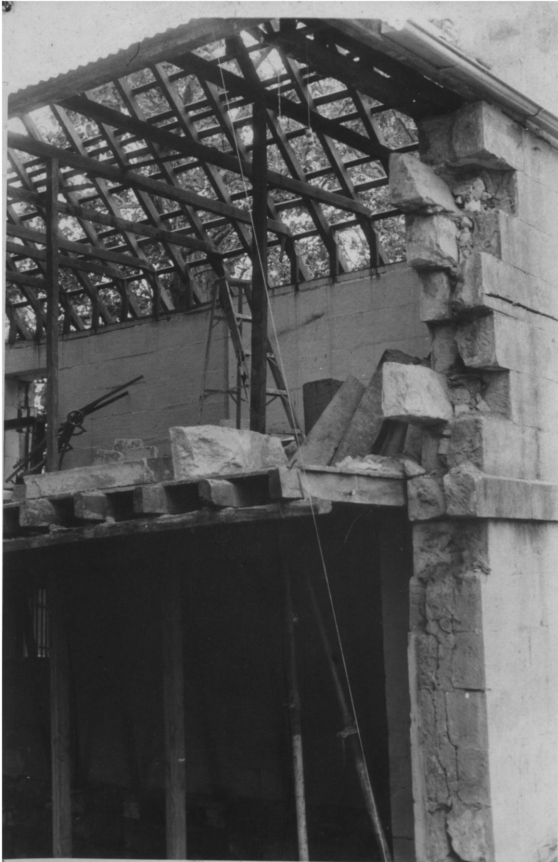
Figure 50 View of north-west corner; South wall and roof structure left intact
