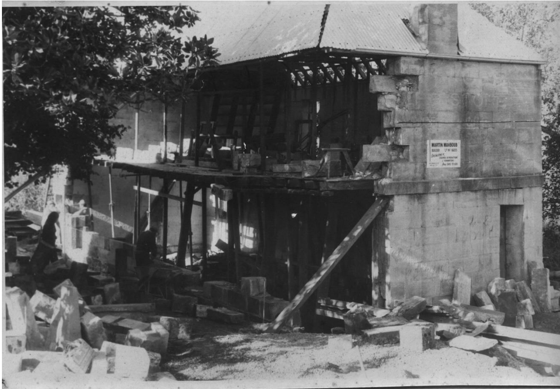
Figure 48 North Wall Dismantled; All blocks numbered
